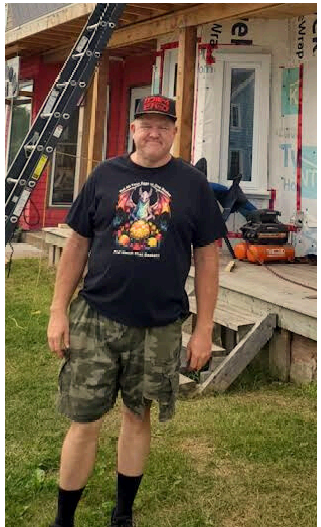
Pic. Briggs in the middle of renovating his Georgetown, P.E.I. home.
